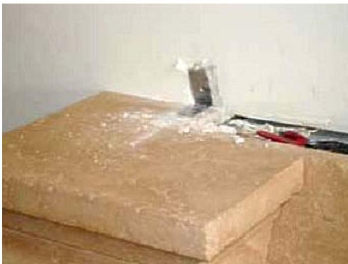
14. Put the Mantel in place to test fit it in the space provided. Properly locate the Mantel per specifications provided in the Installation plan.
