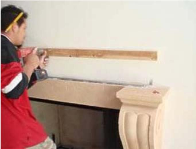
16. Once completed, place the Mantel face down and repeat the bonding methods used in step 8.
